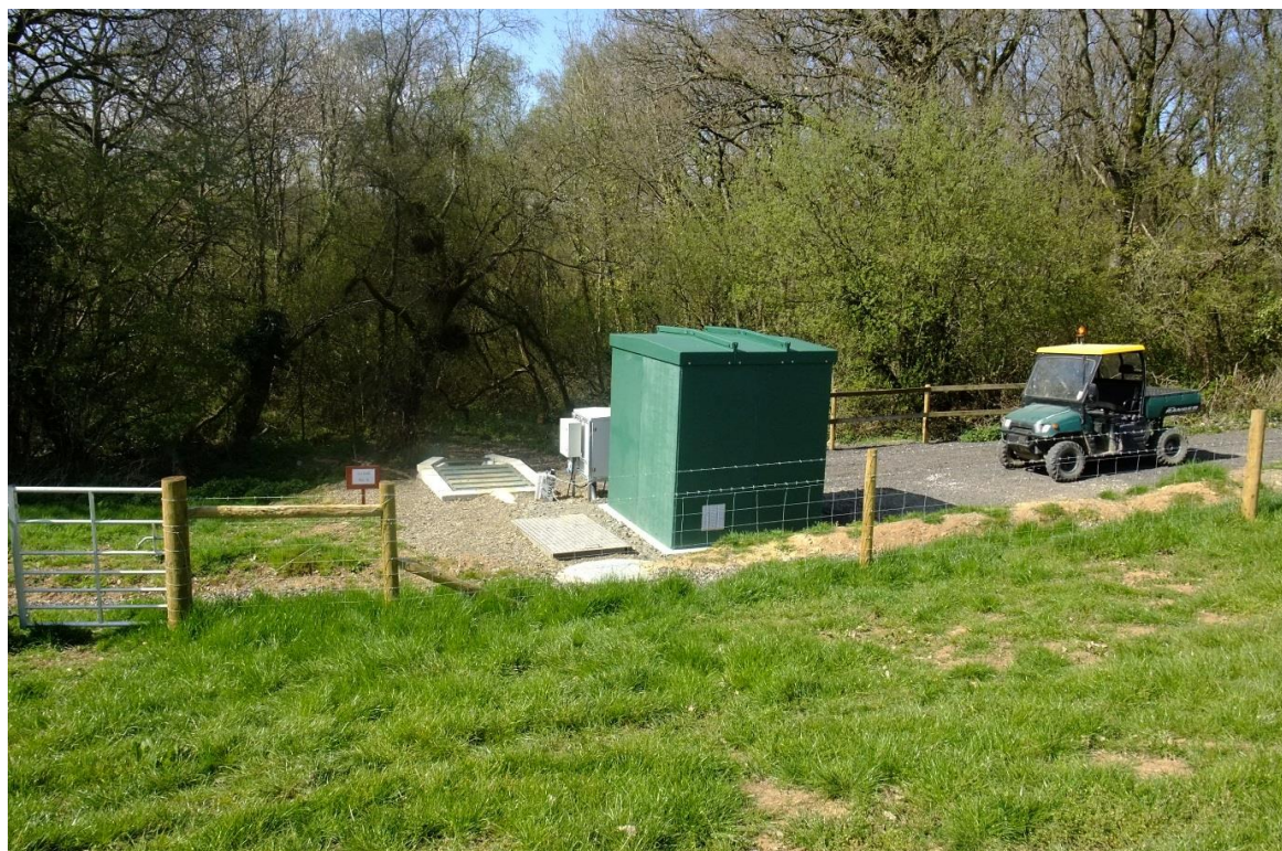
Figure 11. One of fifteen flume laboratories which are sited in each catchment.
