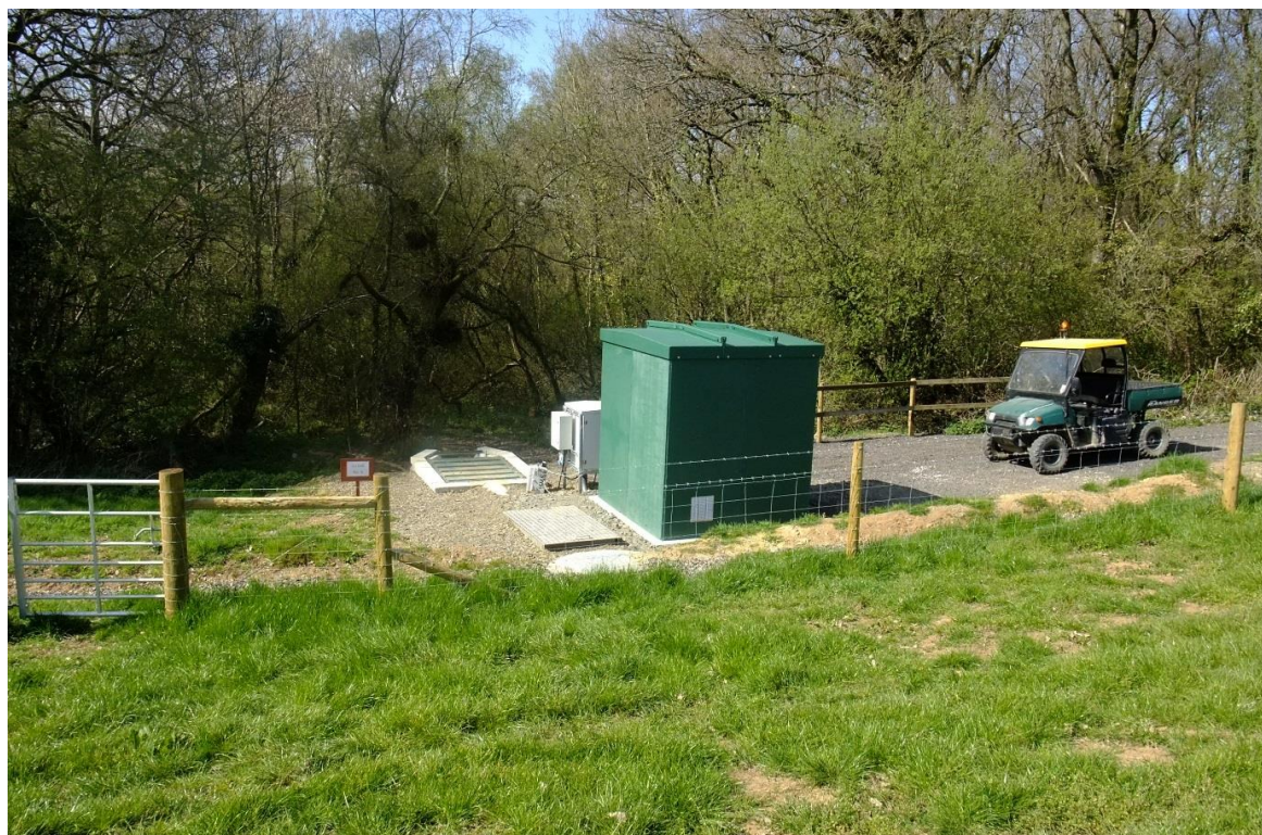
Figure 10. One of fifteen flume laboratories which are sited in each catchment.
