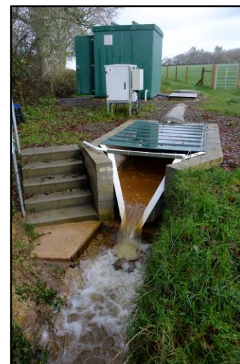
Figure 4. Example of an H-Flume
